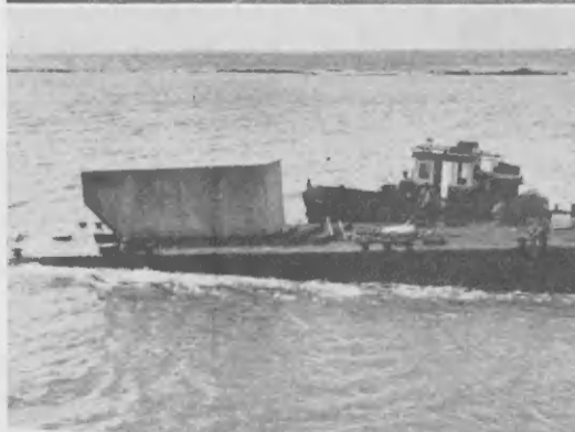
THE QUAY wall, a section of which will be covered with banded concrete slabs, will be 350 meters long. Huge concrete monoliths are fabricated on the site, floated by barge to position and then lowered in place by a floating crane. The Barcadera Harbor has a navigable depth of thirty-six feet.
